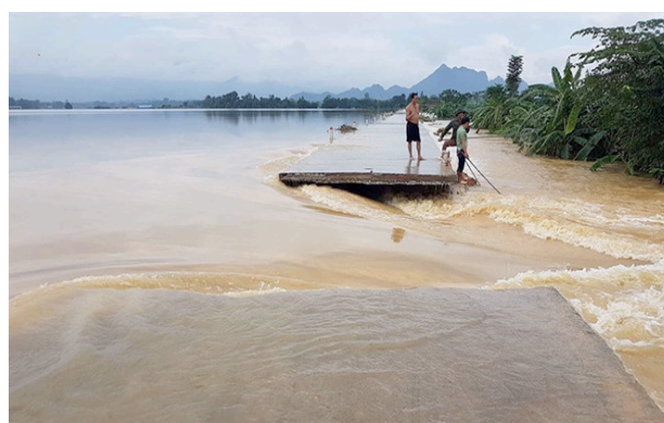
Broken dyke on Bui river in Chuong My district and Xuan Mai town, Ha Noi
